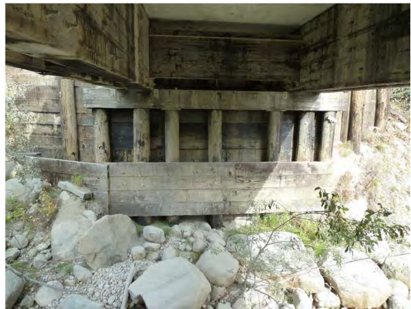
Figure 1-18: Woods end abutment.
