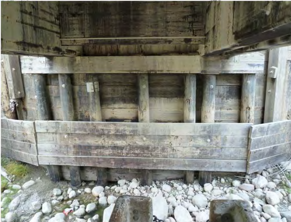
Figure 1-13: Camp end abutment.
