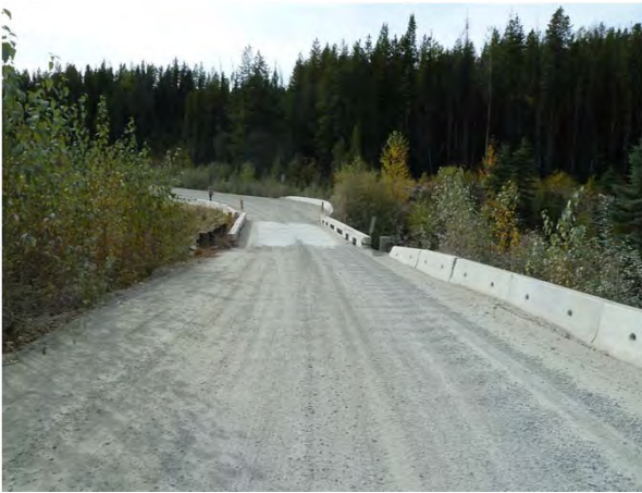
Figure 1-3: Looking towards camp end.
