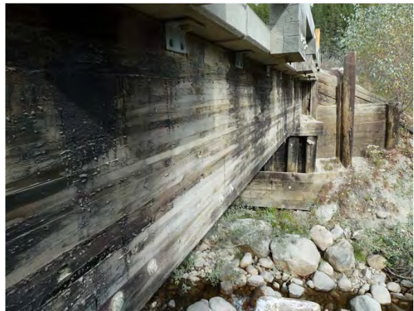
Figure 1-12: Typical downstream face of girder 4.
