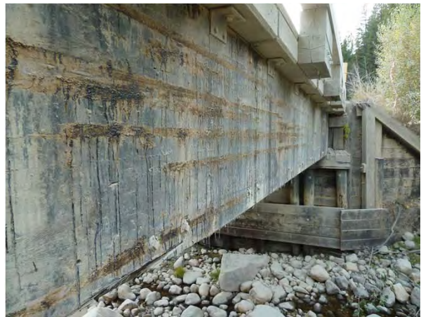
Figure 1-10: Typical upstream face of girder 1.
