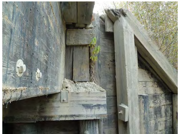
Figure 1-16: Upstream camp end wing wall and abutment.
