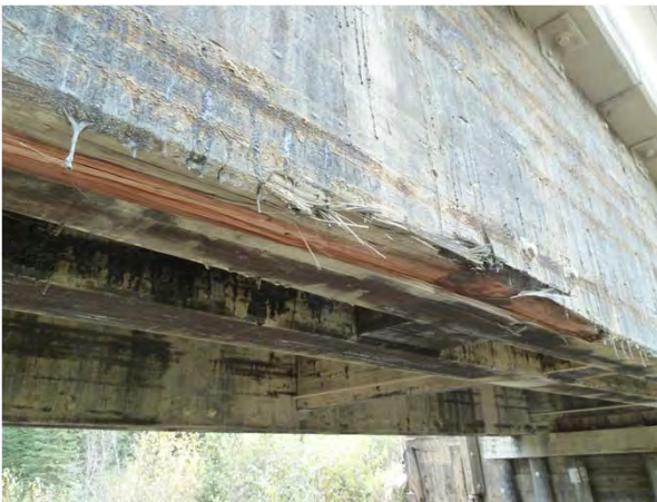
Figure 1-11: Damaged girder 1.
